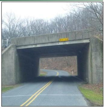
Load posting a bridge is required by the National Bridge Inspection Standards when a bridge is not capable of safely carrying a legal load. If a bridge is deemed deficient, officials will post a maximum load for the bridge. Bridges may be posted for other load-capacity restrictions including speed and number of vehicles permitted on the bridge. There are four (4) load-posted bridges in the area, and all are local-owned.
